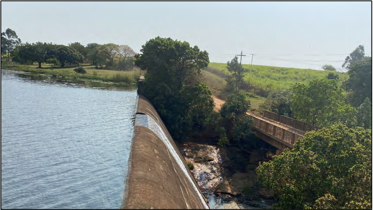
Figure 16.6 Eshlazi Dam (UUW, 2023).
