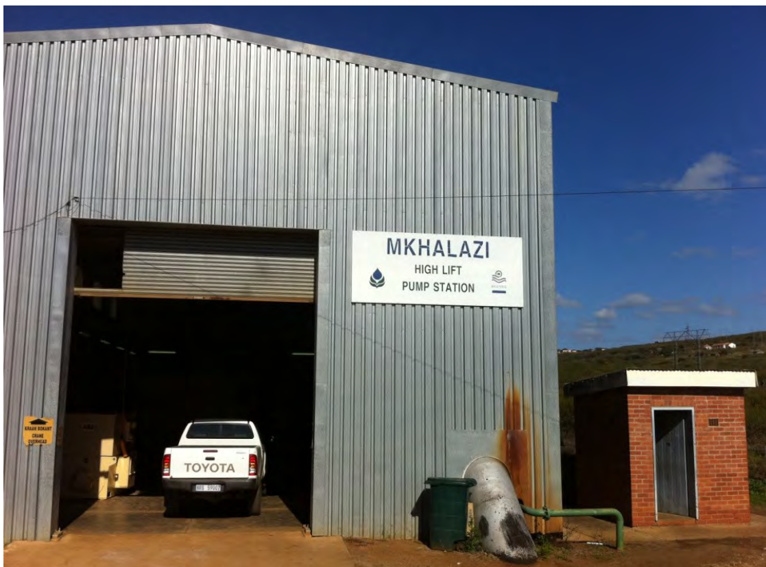
Figure 16.17 The Mkhhalazi High Lift Pump Station.
