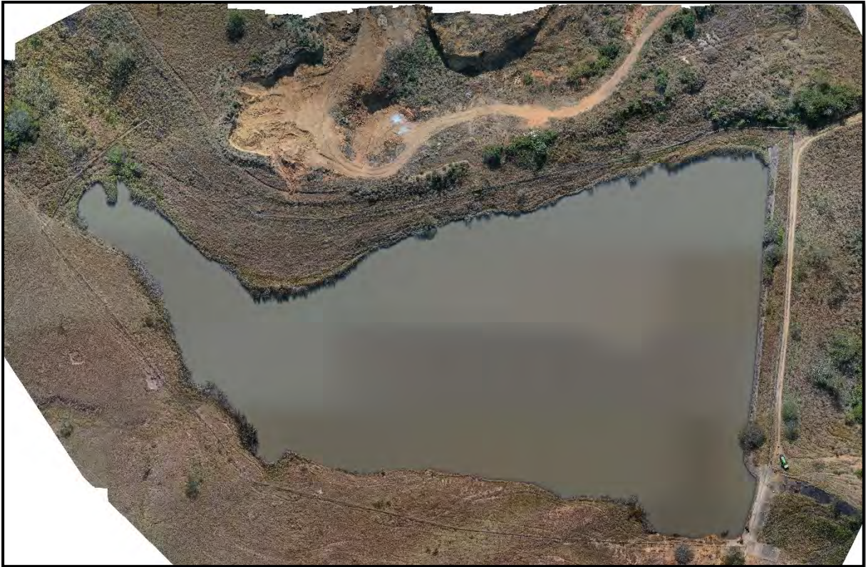
Figure 16.5 Melmoth Off-Channel Storage Dam (UW, 2022).
