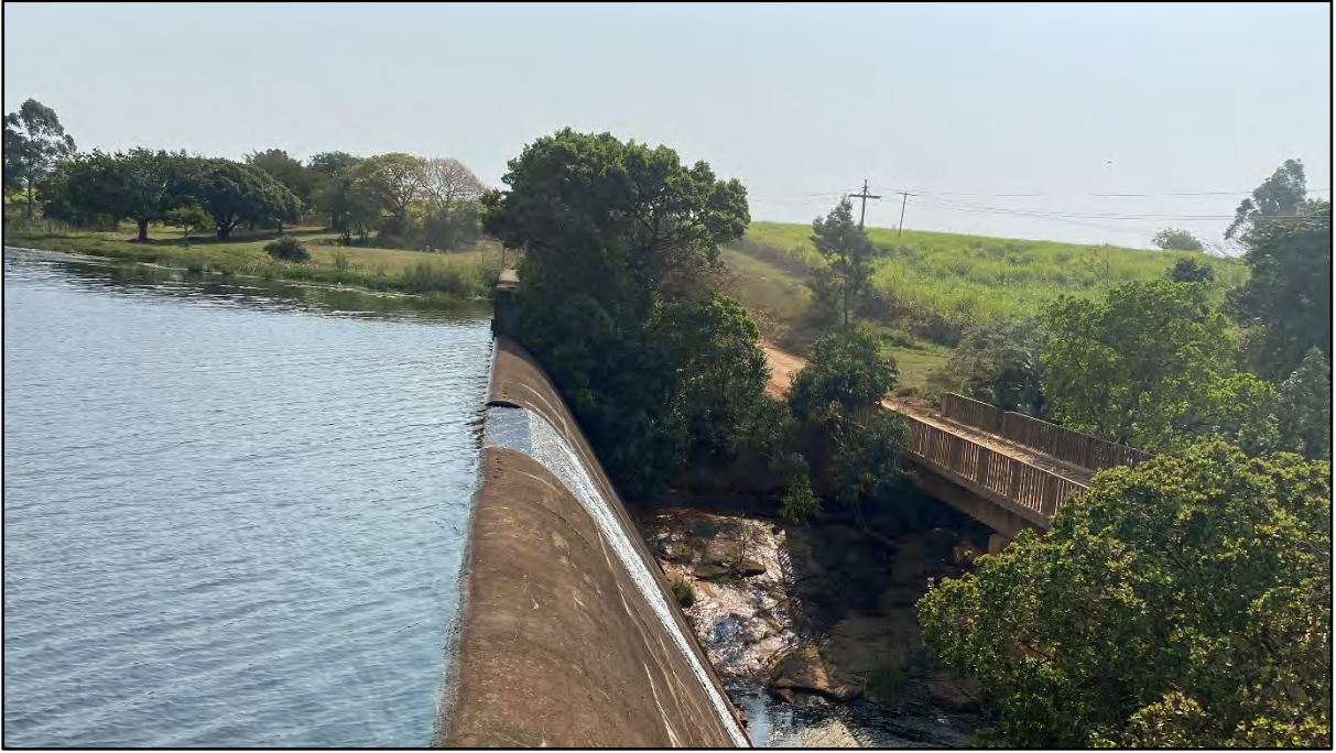
Figure 16.6 Eshlazi Dam (UUW, 2023).
