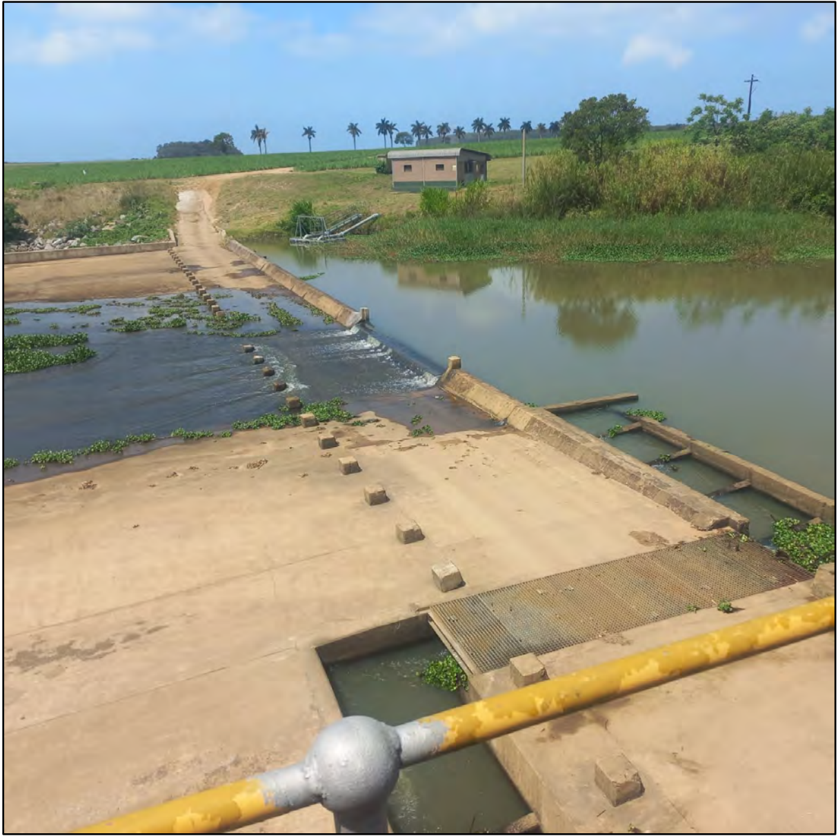
Figure 16.26 uMhlathuze Weir (UUW, 2023).
