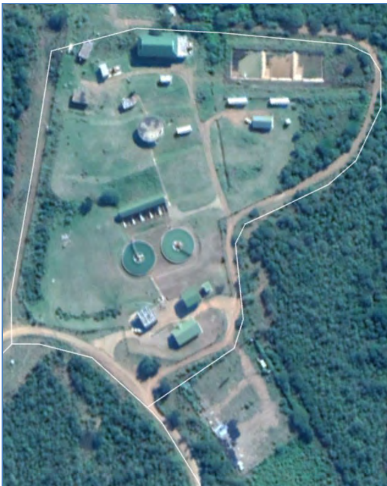
Figure 16.19 Greater Mthonjaneni WTP.
