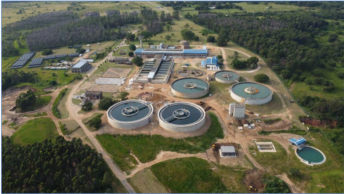
Figure 16.30 Nsezi WTP (Photo taken by UUW, 2025).
