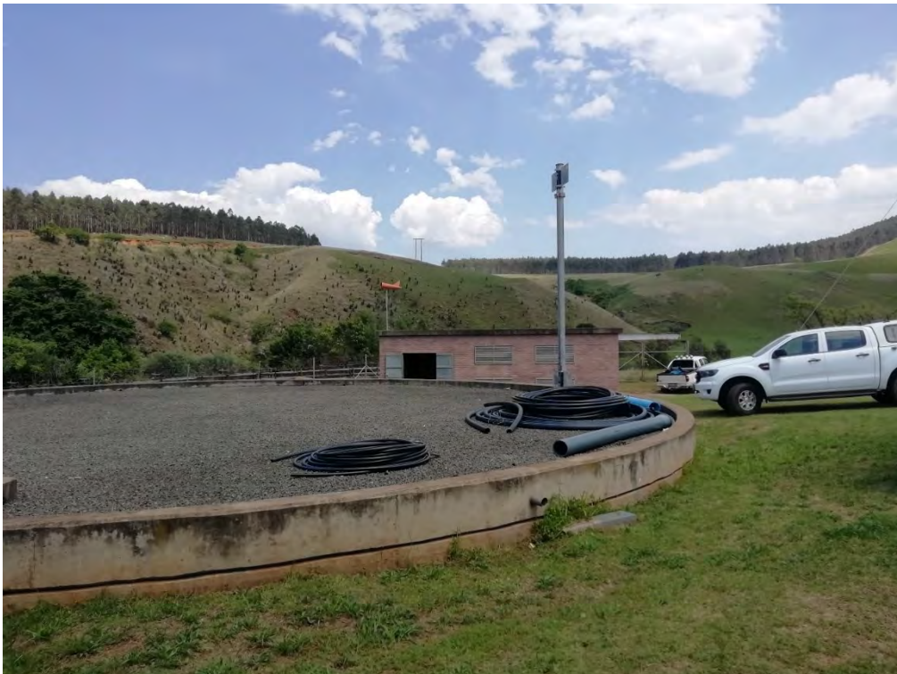
Figure 16.11 The Nkandla WTP (Photo taken by UUW).
