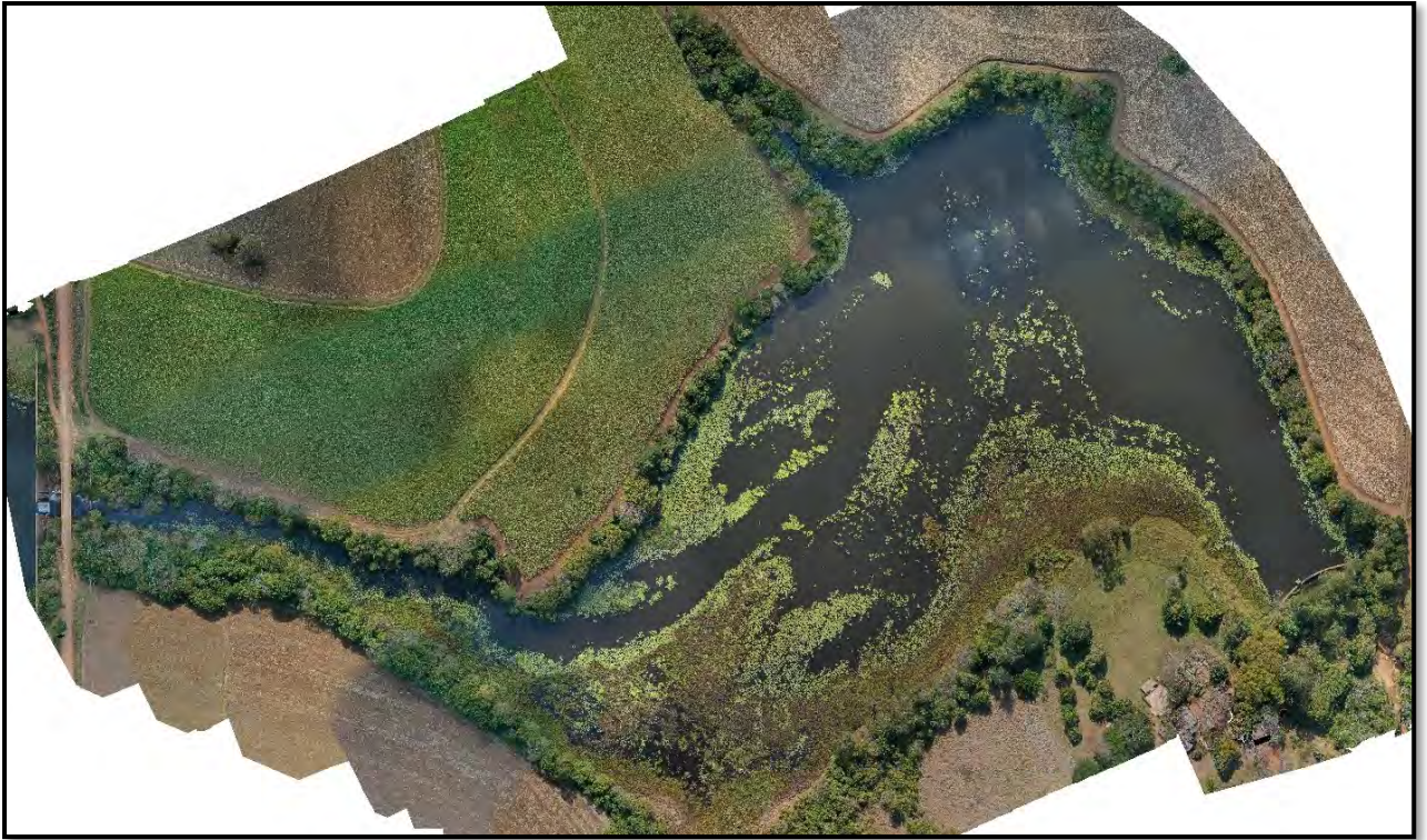
Figure 16.7 Rutledge Park Dam (UUW, 2022).
