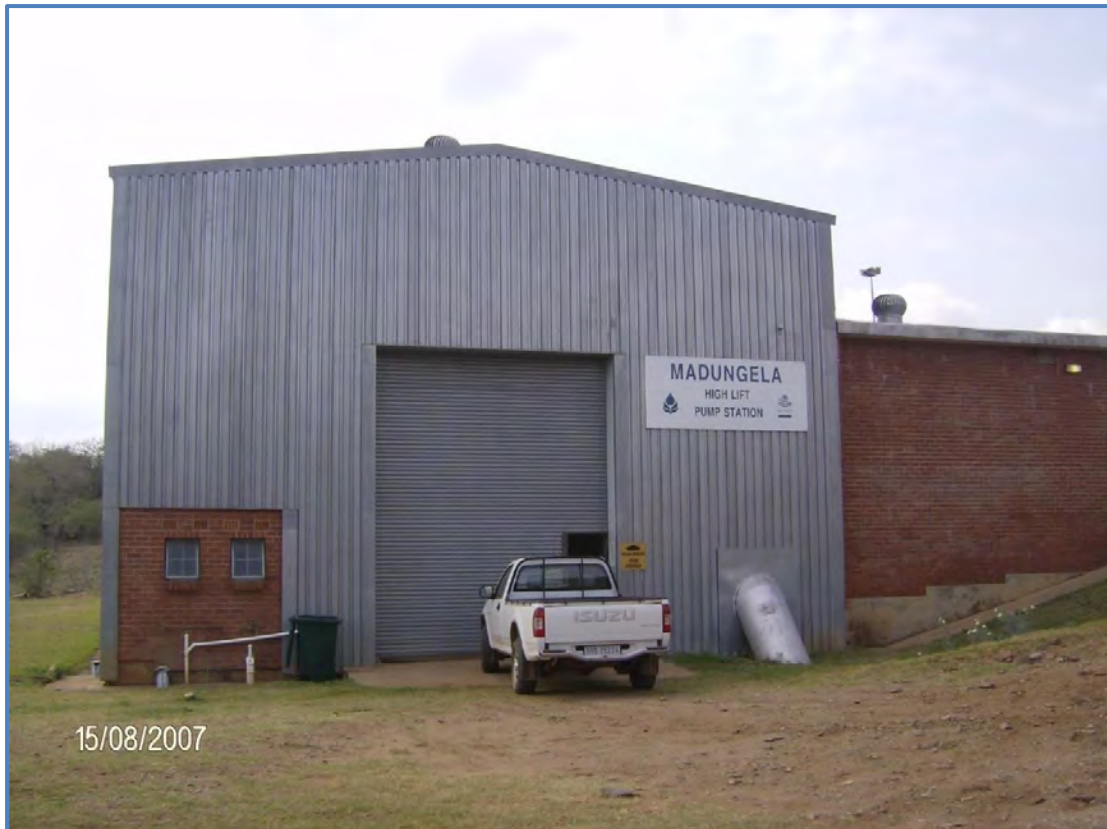
Figure 16.16 The Madungela High Lift Pump Station.
