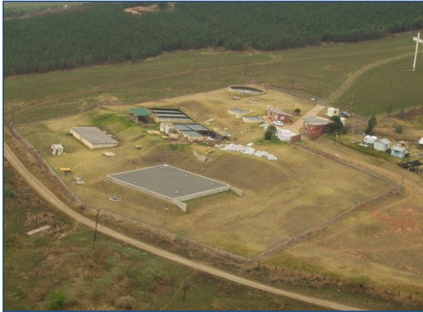
Figure 8.6 Ixopo Water Treatment Plant.
