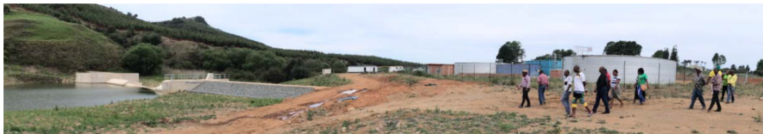
Figure 8.11 Weir and Package Plant on the Luhane River
