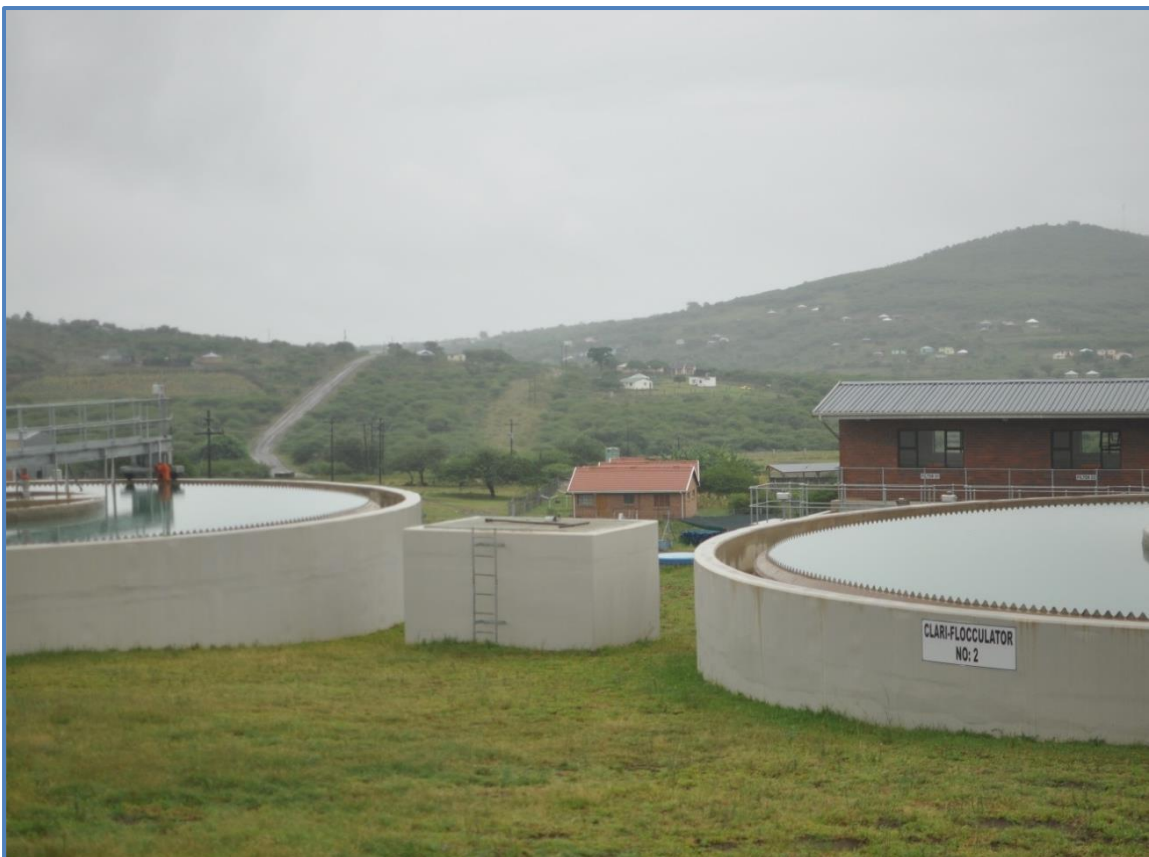
Figure 16.17 Photo of Middledrift WTP Clarifiers.
