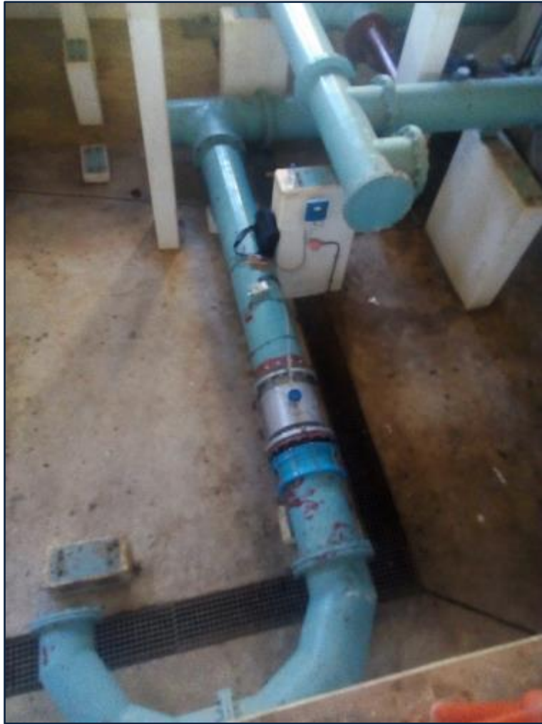
Figure 13.47 Ekuvukeni sales meter (Umgeni Water 2019).
