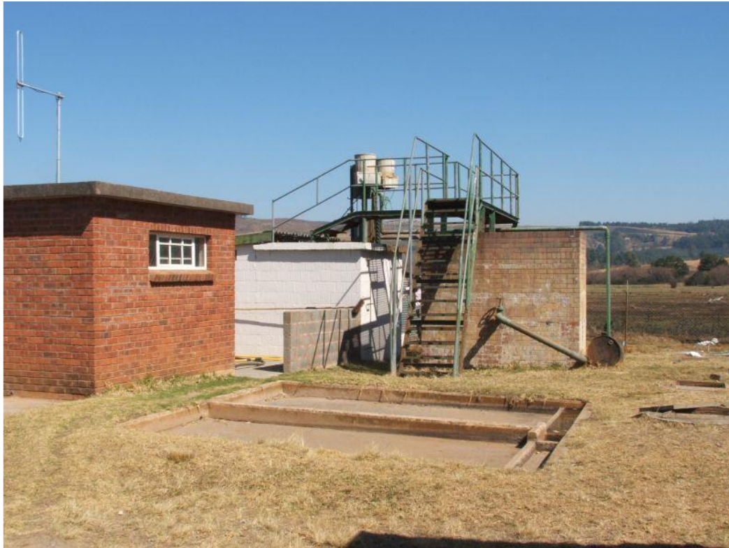
Figure 7.75 Lidgetton WTP sand wash bays with old dosing system (uMgungundlovu District Municipality 2010)
