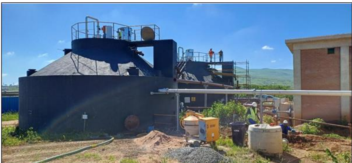
Figure 19.119 Anaerobic Digesters pipework being connected.
