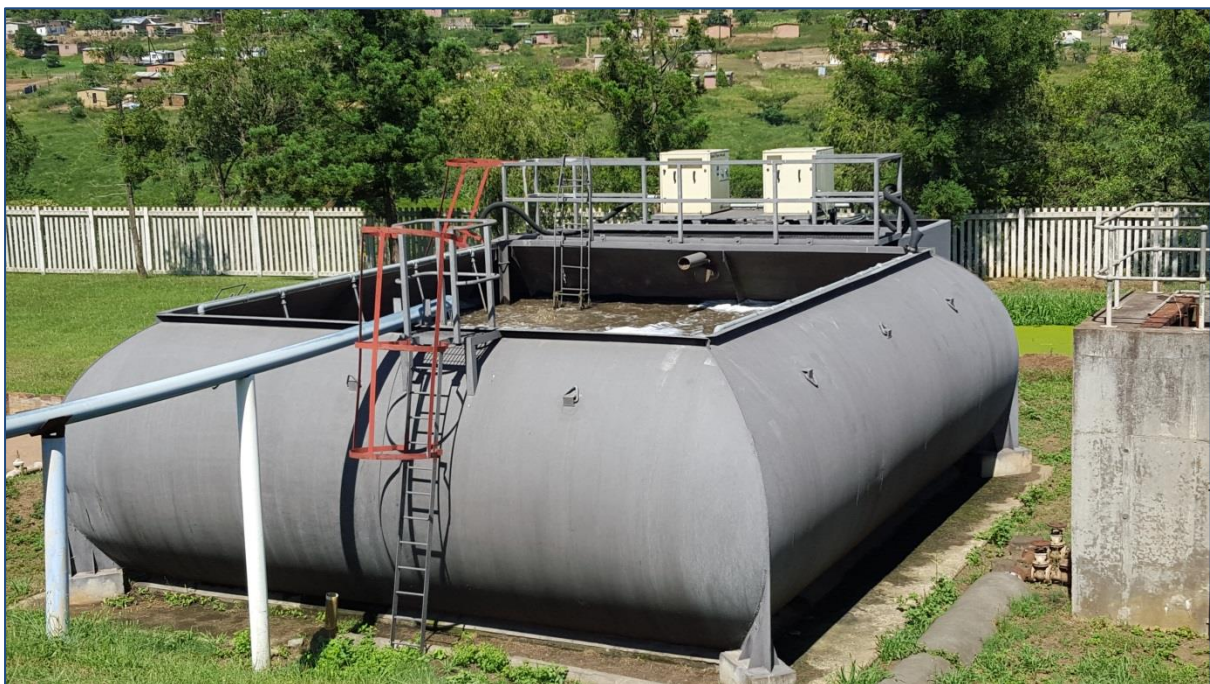
Figure 19.18 Sequencing Batch Reactor (SBR) Albert Falls North WWW.
