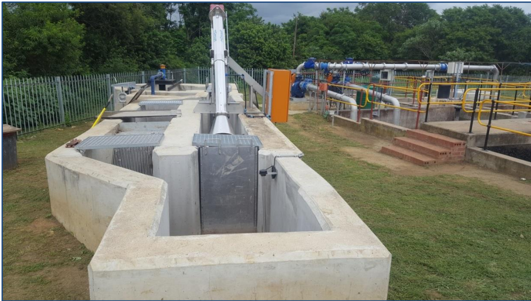
Figure 19.36 Lynnfield Park WWW head of works showing manual and mechanical screening channels.
