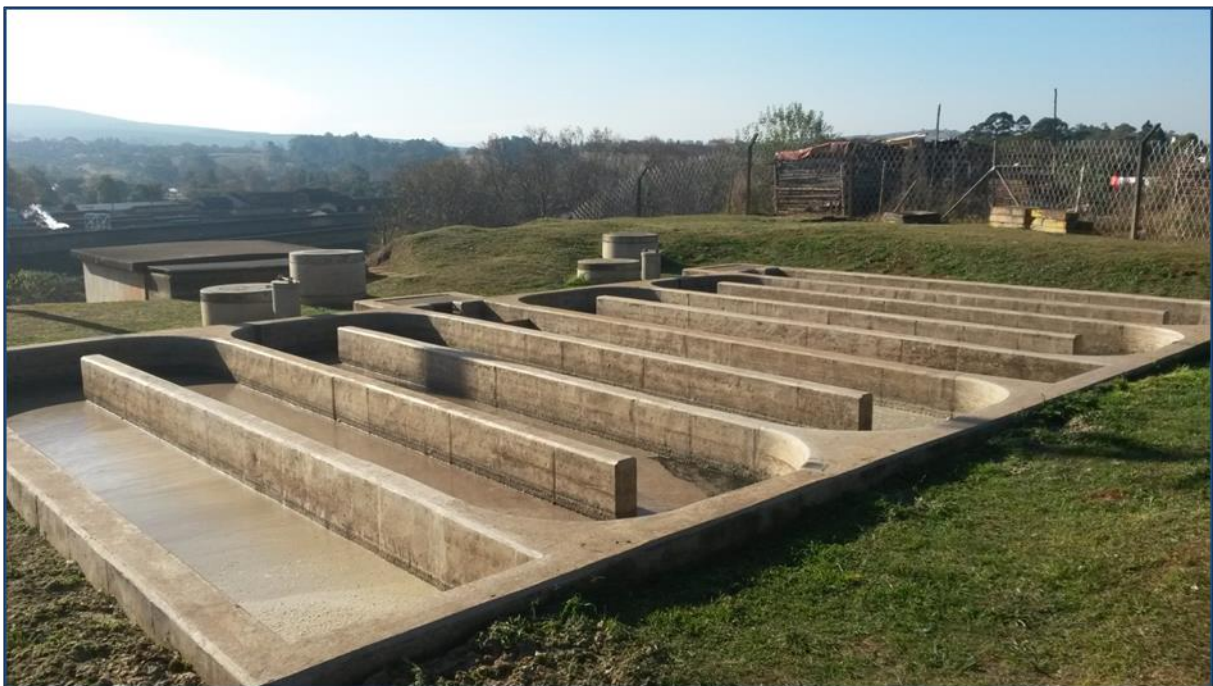
Figure 19.27 Howick WWW Chlorine Contact Tank.
