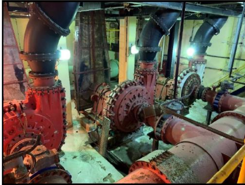
Figure 19.25 Alkantstrand B-Line pump sets (not operational) (Mhlathuze Water 2022: 53).
