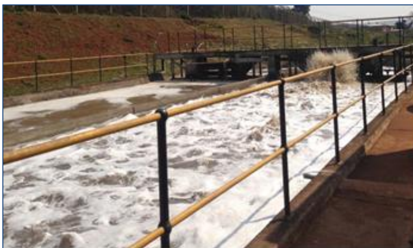
Figure 19.50 Appelsbosch WWW Oxidation Ditch (Aeration Tank).
