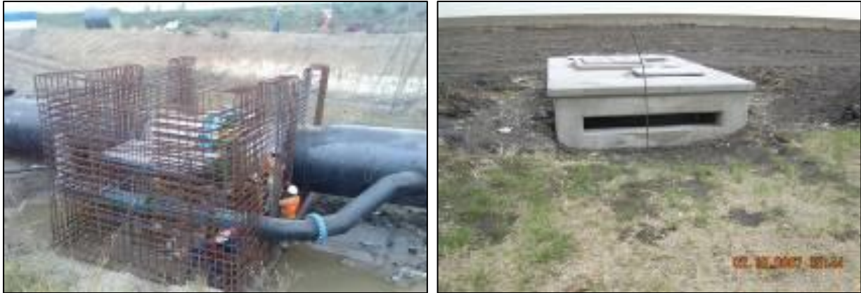
Figure 12: Typical examples of chambers (left - during construction; right – completed)
