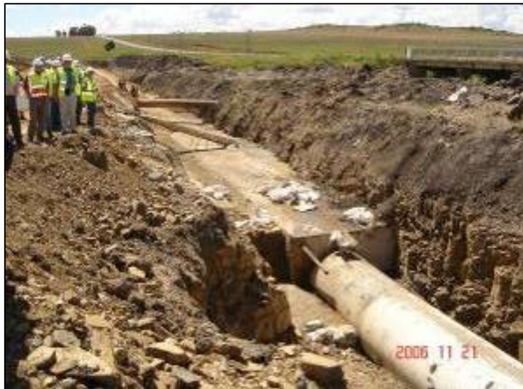
Figure 14: Typical river crossing showing concrete encased pipe section
