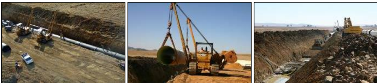
Figure 11: Typical trench excavation and pipe installation activities
