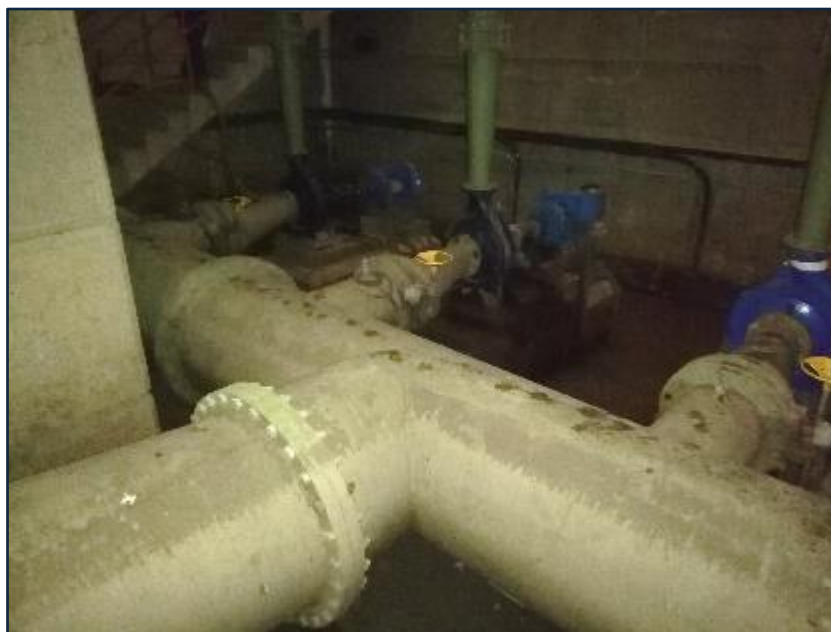
Figure 13.41 Olifantskop raw water pumps (uMngeni-uThukela Water 2019).
