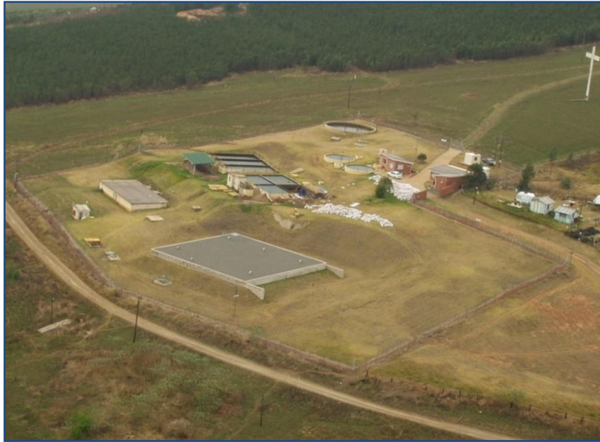
Figure 8.5 Ixopo Water Treatment Plant.
