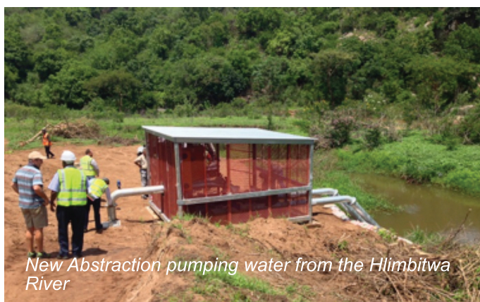
Outlet pipe discharges water from Hlimbitwa into existing abstraction works
