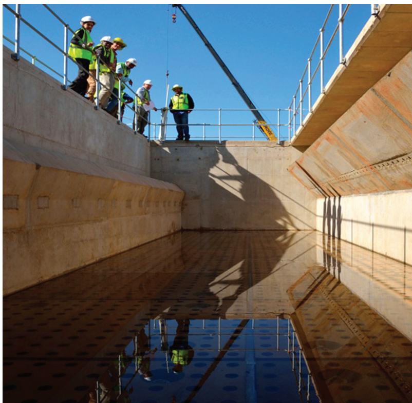
Members of the Design and Construction team look on during a filter level test.
