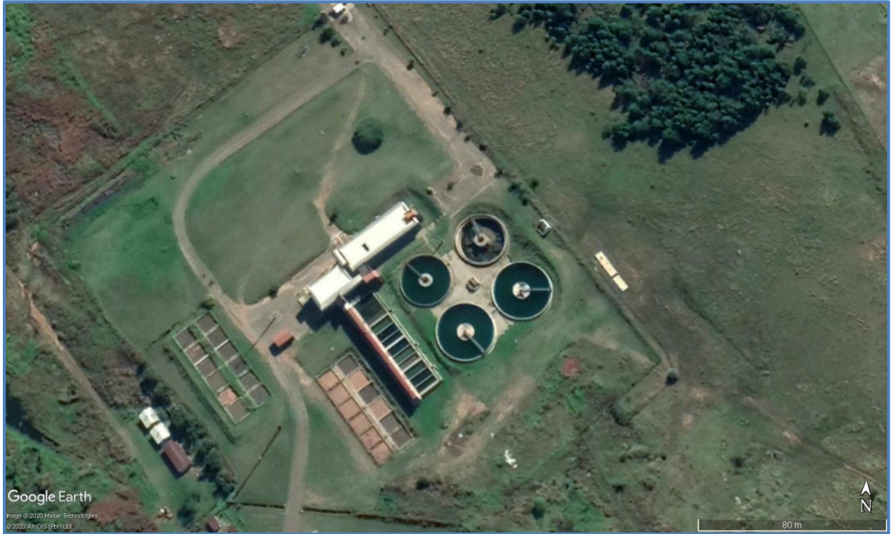
Figure 17.26 An Aerial view of the Klipfontein WTP
