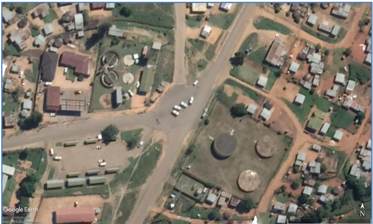
Figure 18.21 Aerial view of Frischgewaagd Water Treatment Plant
