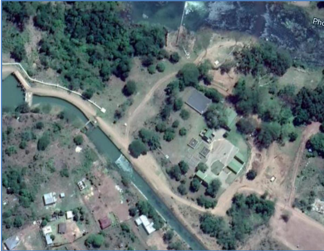
Figure 18.36 Aerial view of Jozini New Water Treatment Plant
