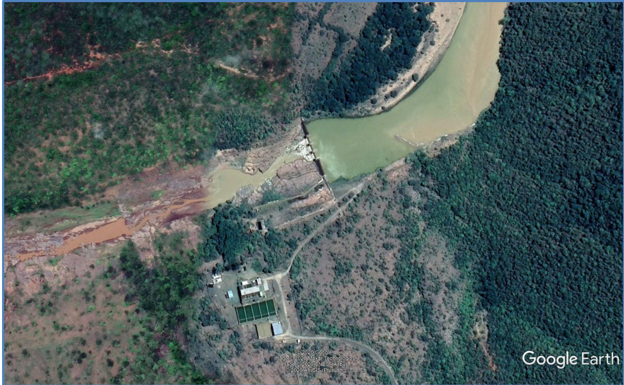
Figure 17.15 Aerial view of the weir and Ulundi Water Treatment Plant
