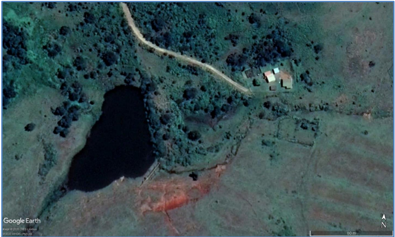
Figure 17.16 Aerial view of the Nkonjeni Dam and Nkonjeni Water Treatment Plant
