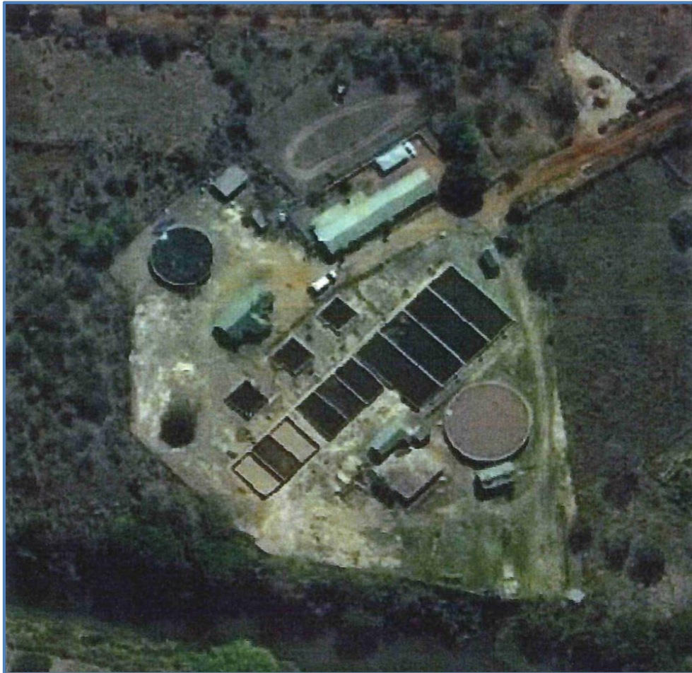
Figure 18.40 Aerial view of the Shemula (Old) WTP
