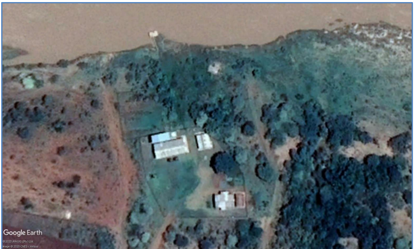
Figure 17.21 An Aerial view of the Mpungamhlope WTP
