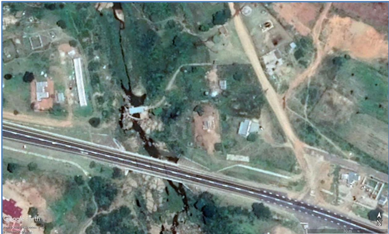
Figure 18.25 Aerial view of Spekboom Water Treatment Plant
