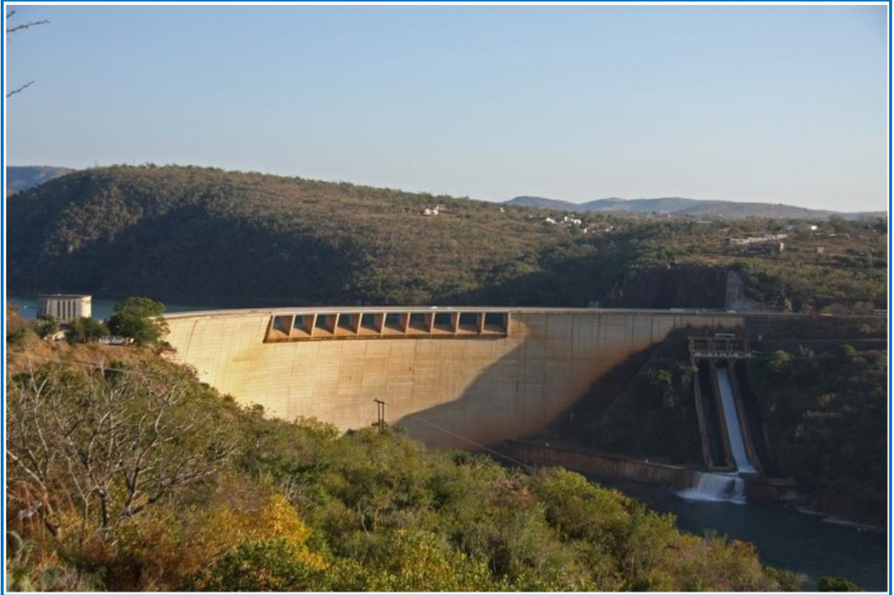
Figure 18.9 Pongolapoort Dam – Source ( https://www.royaljozini.com/pongolapoort-dam-some-history/ )
