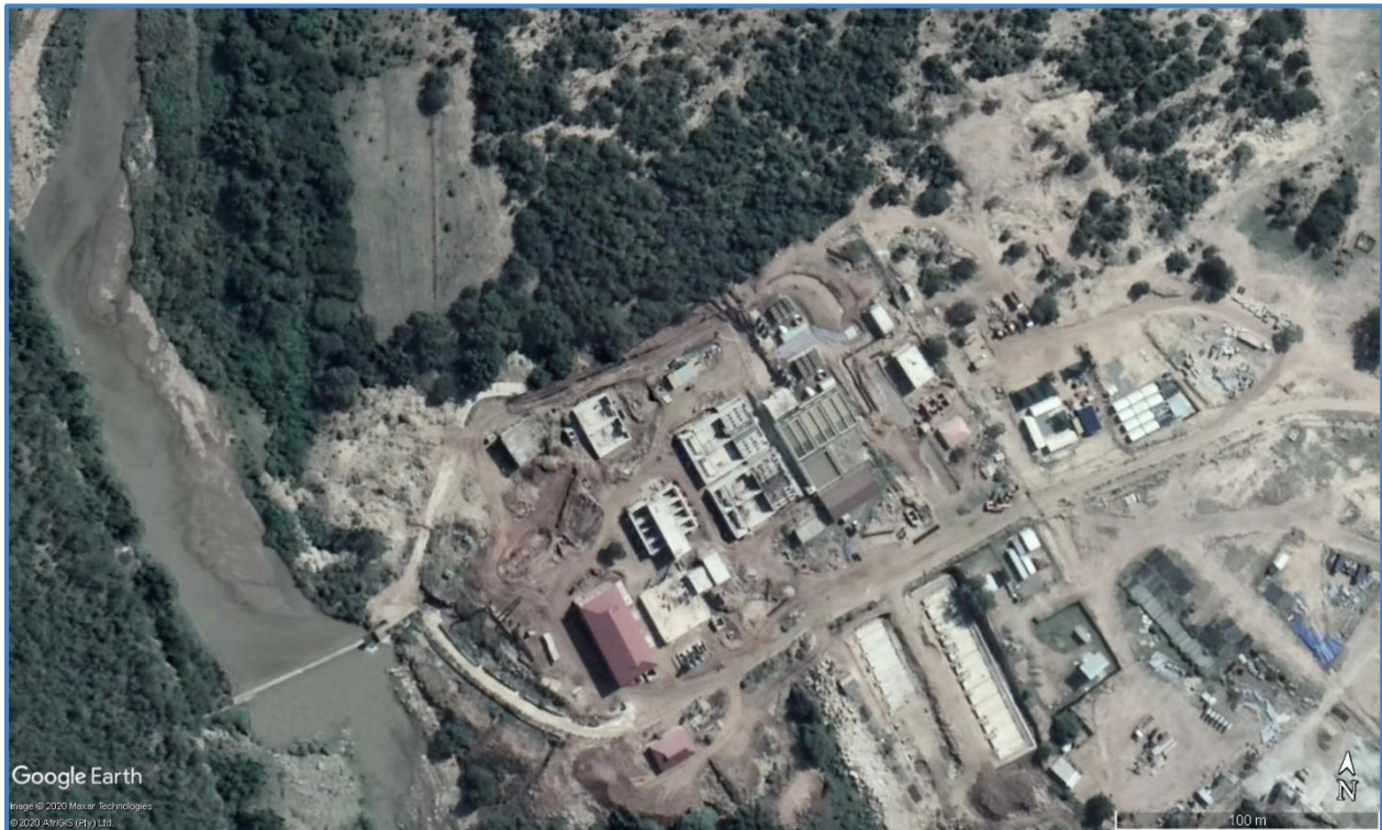
Figure 17.23 An Aerial view of the Usuthu WTP
