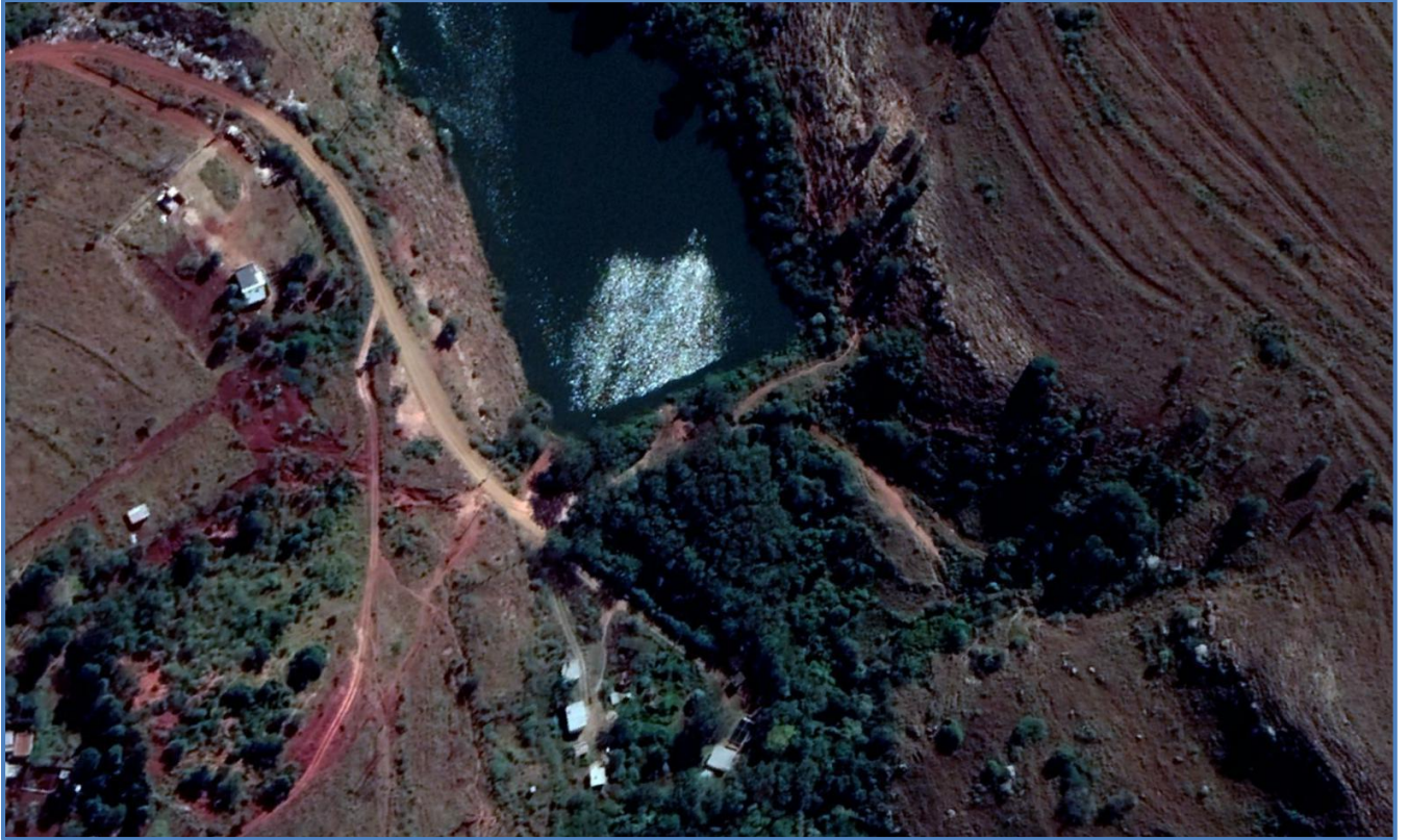
Figure 17.19 An Aerial view of the Embile WTP and the Embile Dam
