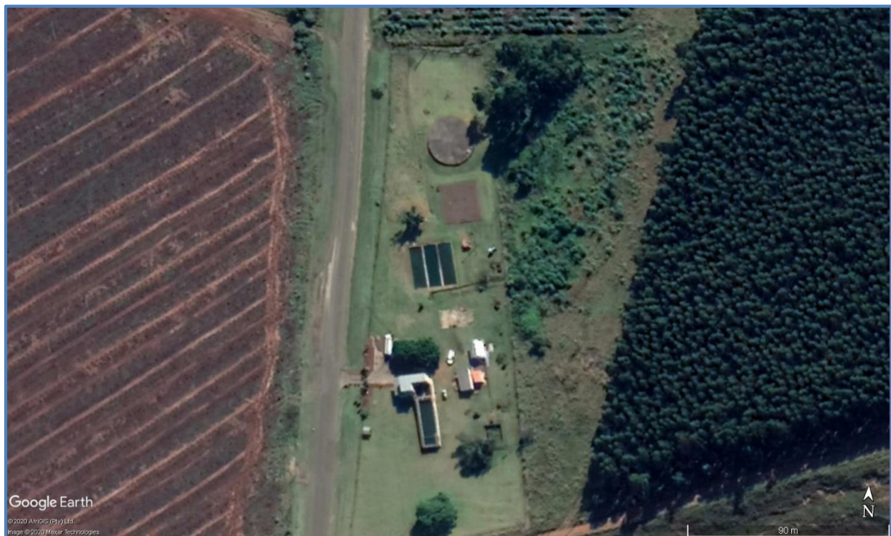
Figure 18.19 Aerial view of Edumbe Water Treatment Plant
