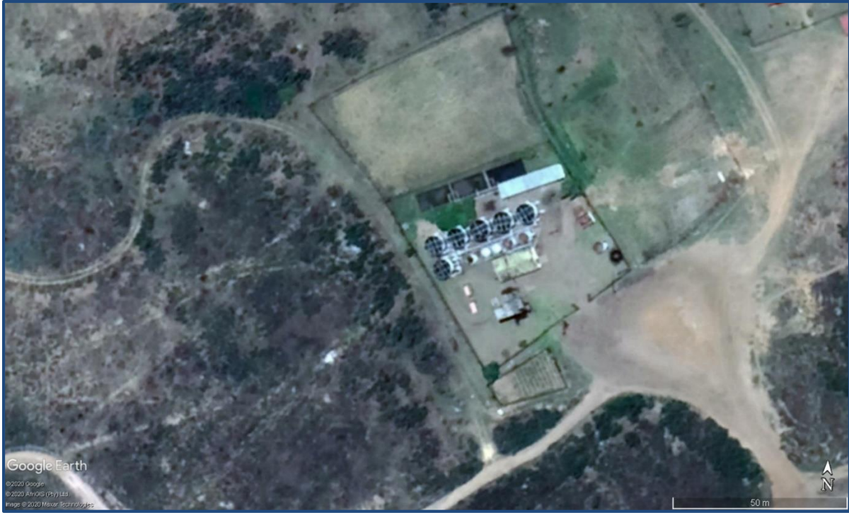
Figure 18.14 Aerial View of the Hlobane WTP
