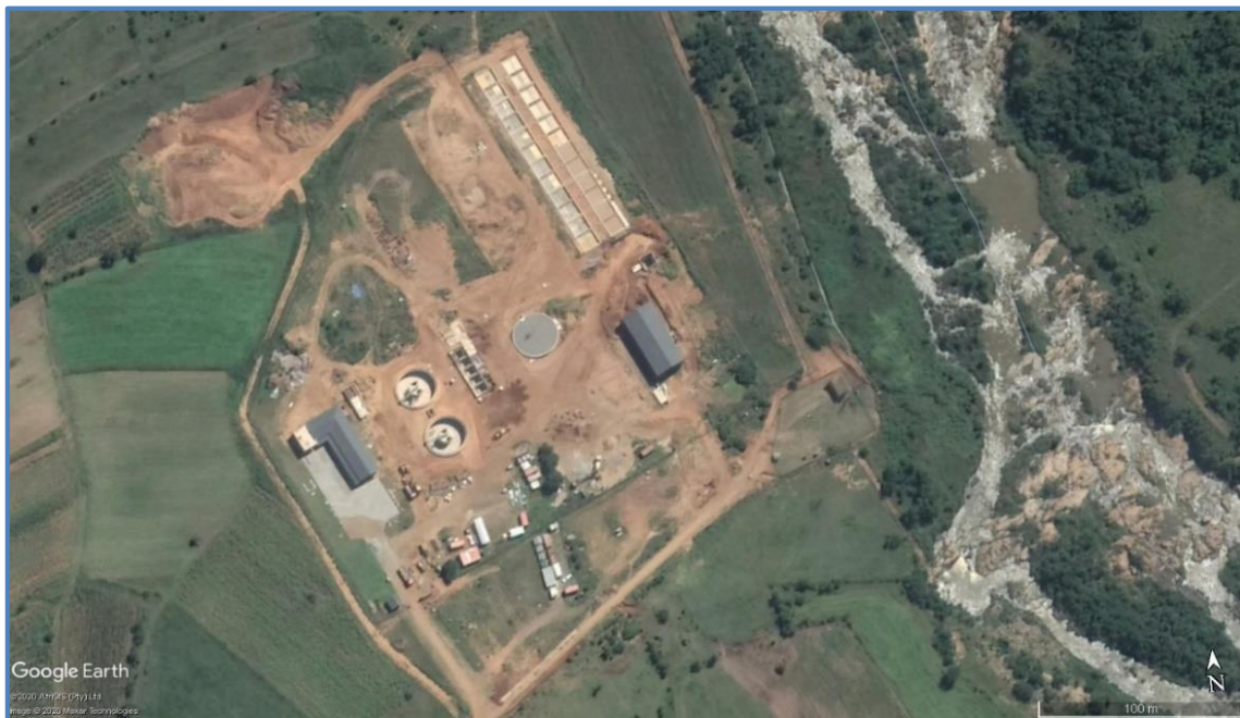
Figure 18.43 Construction of new 15 Mℓ/day WTP at Frischgewaagd along the Phongola River
