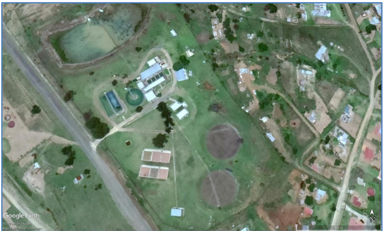
Figure 17.28 An Aerial view of the Mondlo WTP
