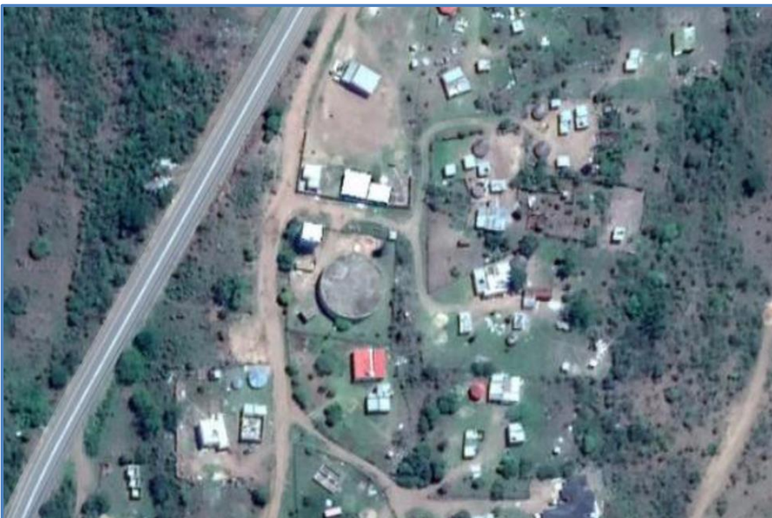
Figure 18.37 Aerial view of Jozini Reservoir
