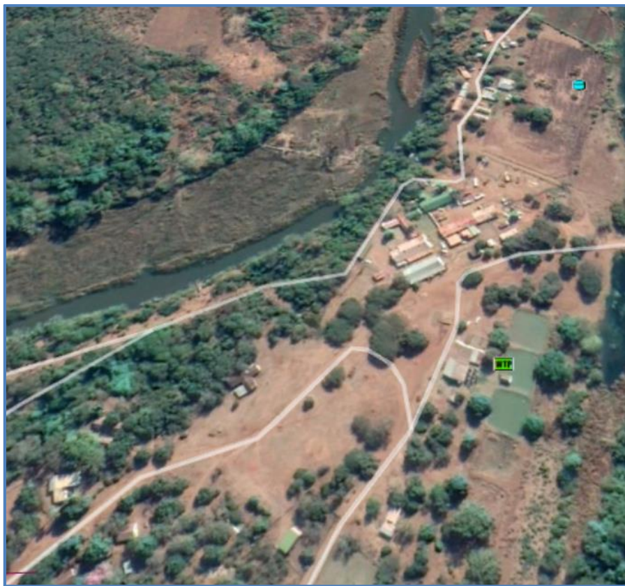
Figure 18.29 Aerial view of Mjindi Water Treatment Plant
