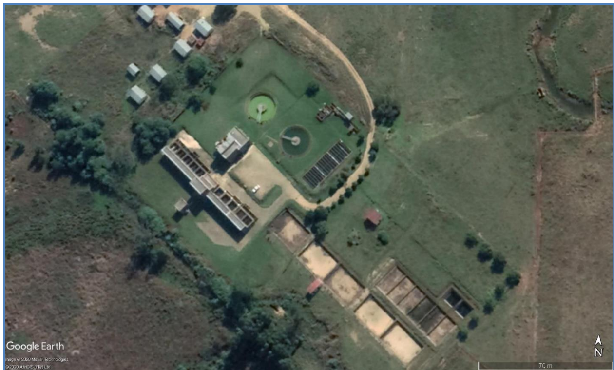
Figure 17.25 An Aerial view of the Bloemveld WTP
