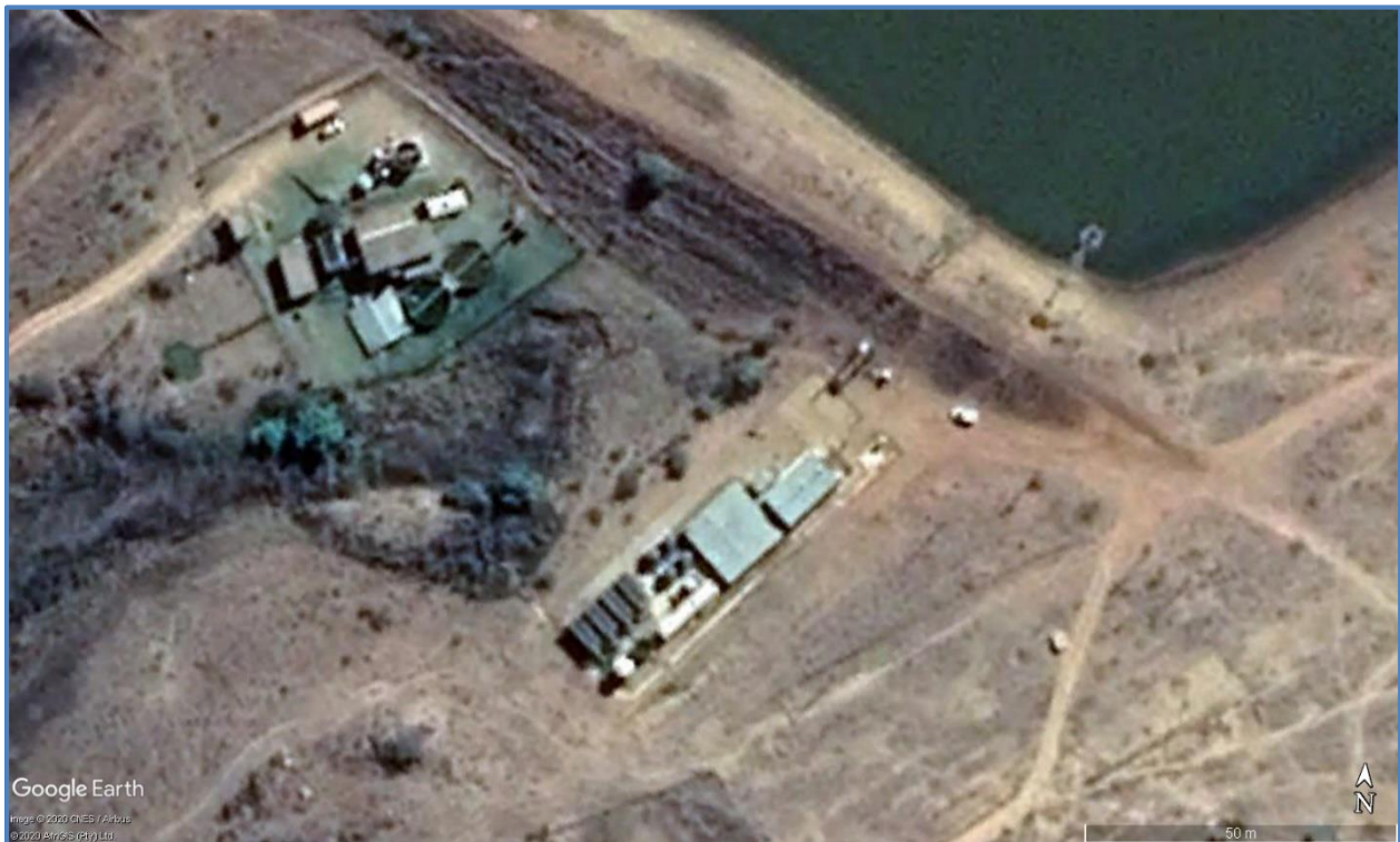
Figure 18.23 Aerial view of Belgrade Water Treatment Plant
