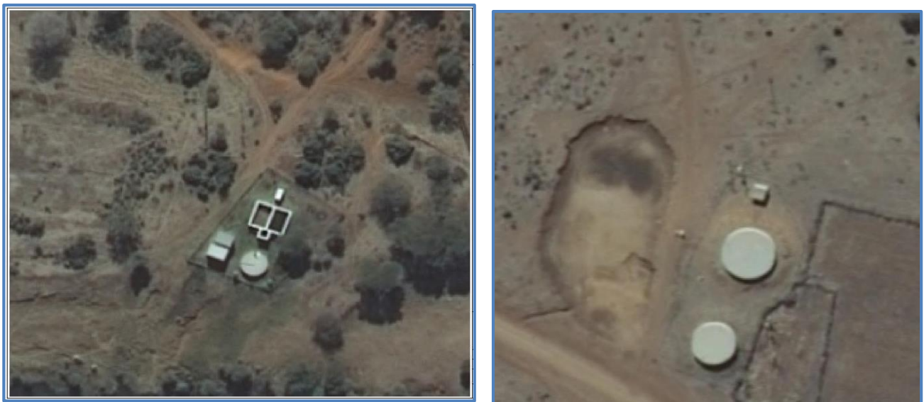
Figure 18.31 Aerial view of Nondebuya Water Treatment Plant & Nondabuya Reservoirs
