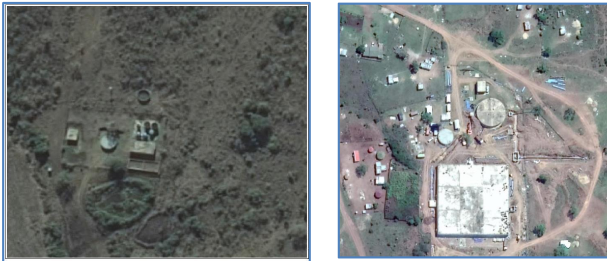
Figure 18.33 shows an aerial view of the Othobothini WTP
