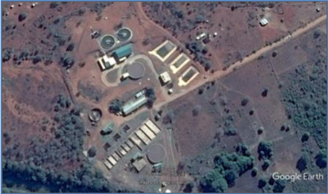
Figure 18.41 Aerial view of Shemula New Water Treatment Plant
