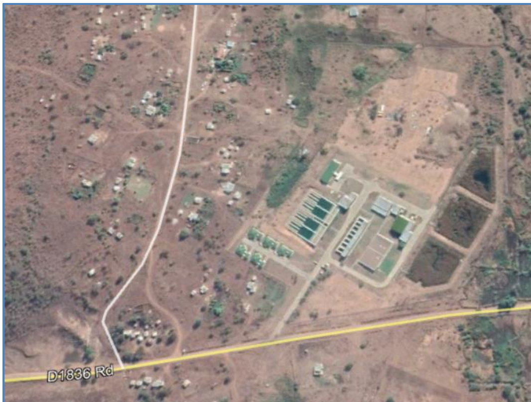
Figure 18.44 Aerial view of Regional Water Treatment Plant (NEW)
