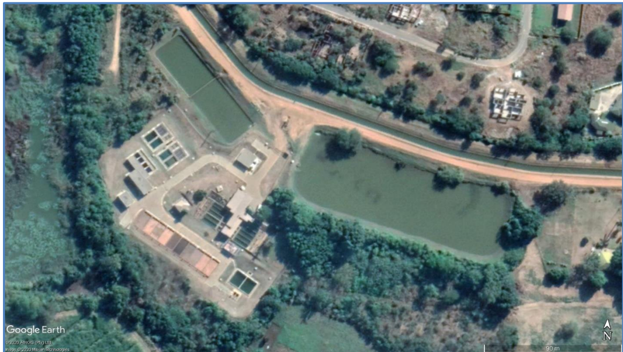
Figure 18.27 Aerial view of Phongola Water Treatment Plant
