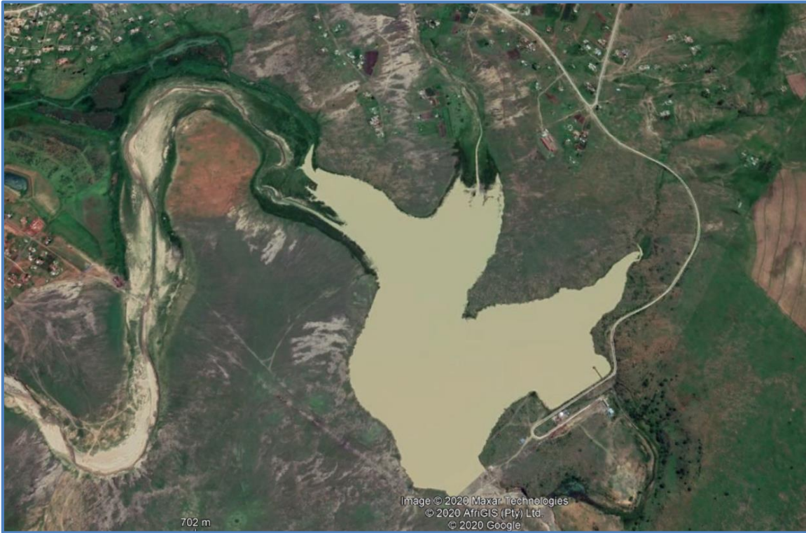
Figure 17.9 Mvunyana Dam (Goole Photo: 2020)
