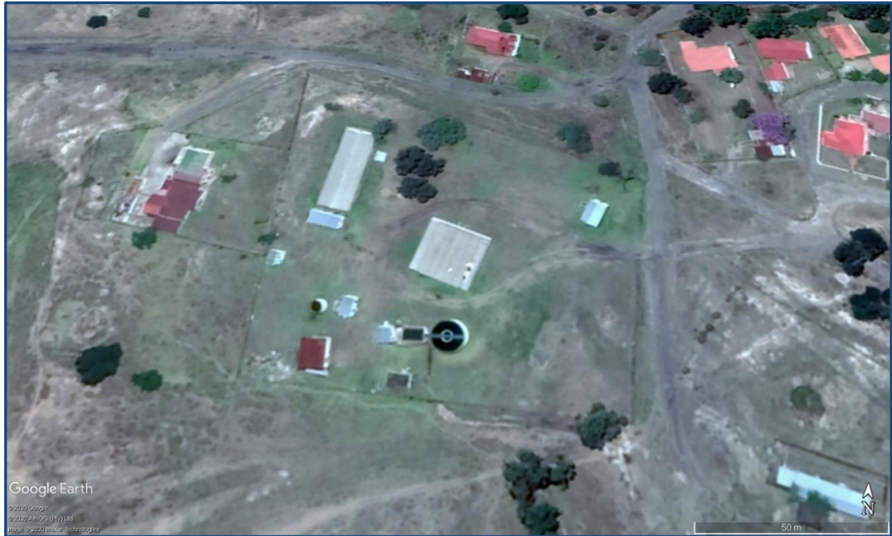
Figure 18.16 Aerial view of Coronation WTP
