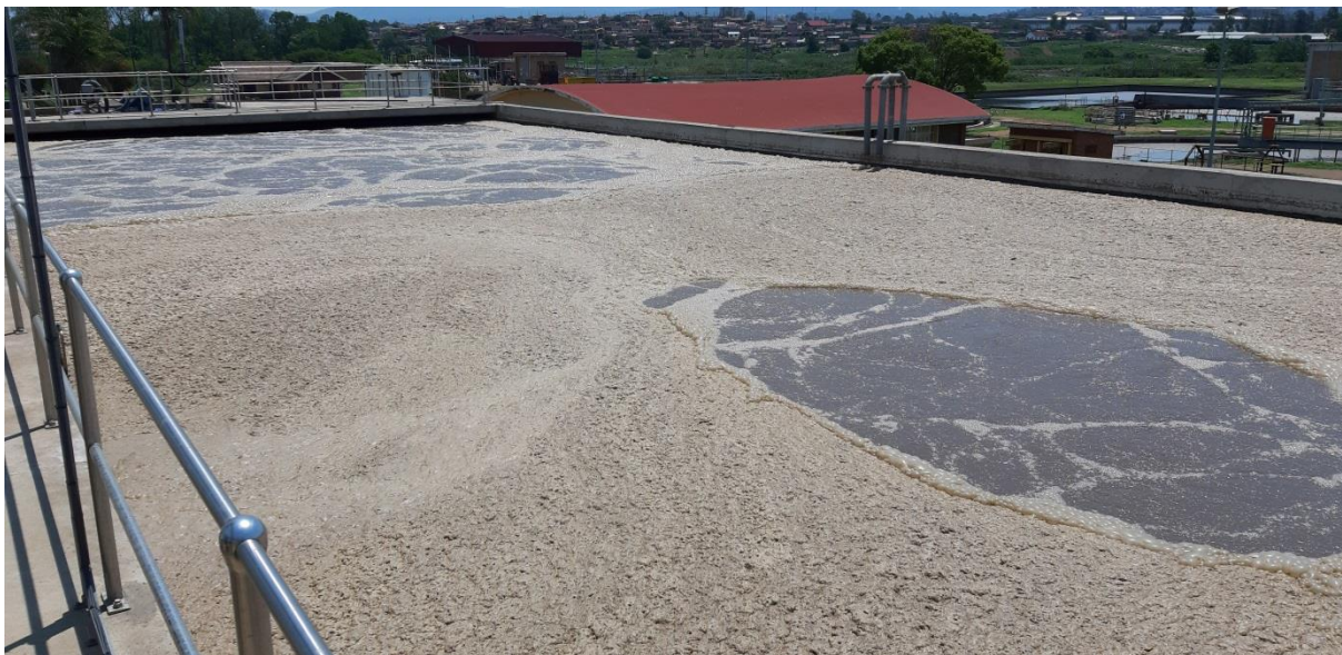
Figure 19.7 Darvill Aeration Basin.
