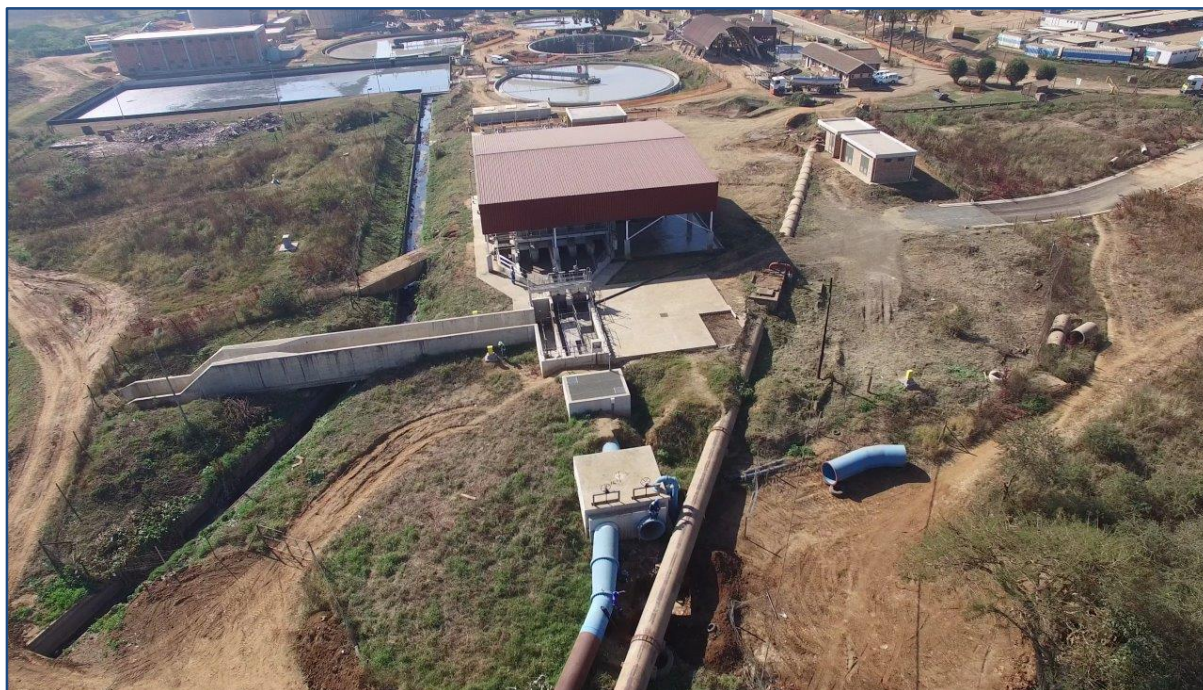
Figure 19.41 New head of works in the foreground with overflow channel teeing-off to the left.
