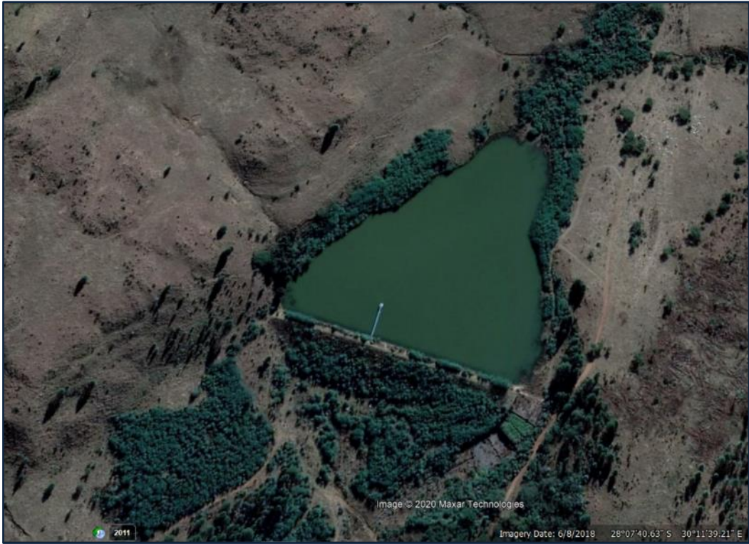
Figure 14.16 Upper Mpate Dam (Google Earth 2018: website).
