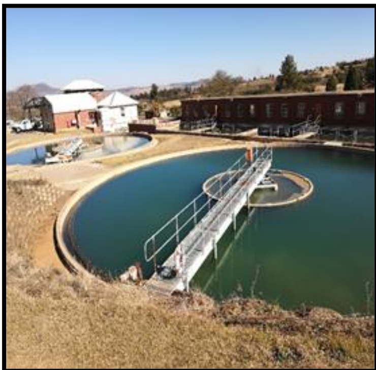
Figure 14.24 Photo of Biggarsberg WTP, Clarifiers (July 2019)
