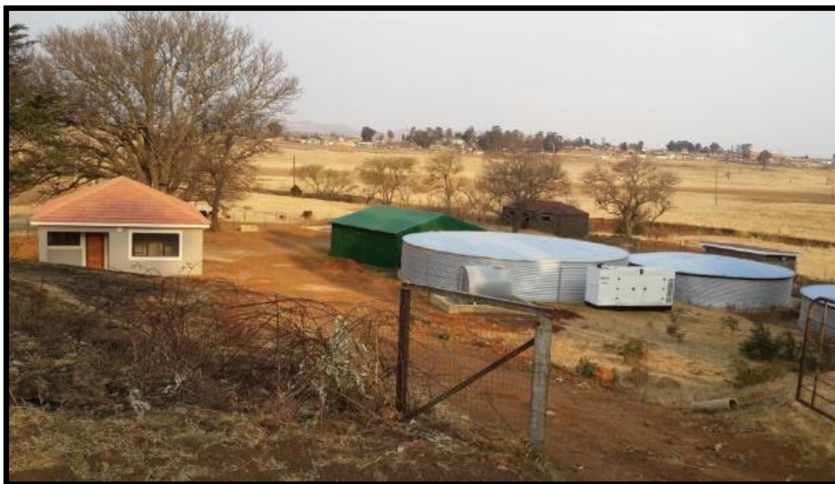
Figure 14.43 Photo of Charlestown Water Treatment Plant (July 2018).
