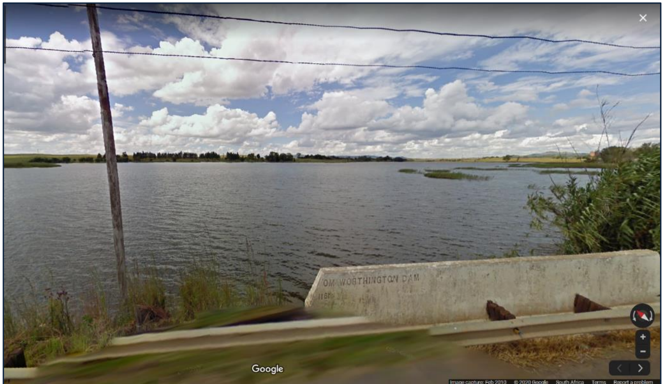
Figure 14.12 Tom Worthington Dam (Google StreetView 2010: website).
