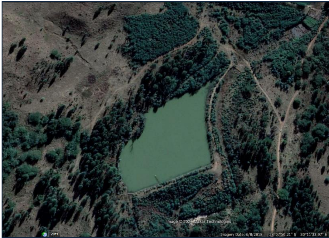
Figure 14.17 Lower M pate Dam (Google Earth 2018: website).
