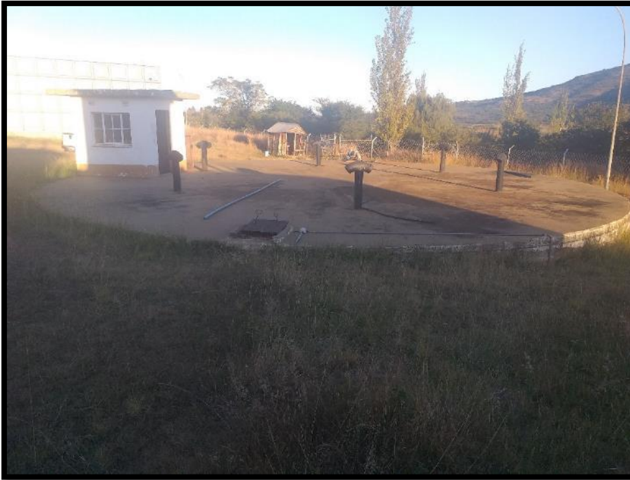
Figure 14.42 Utrecht Clear water Reservoir
