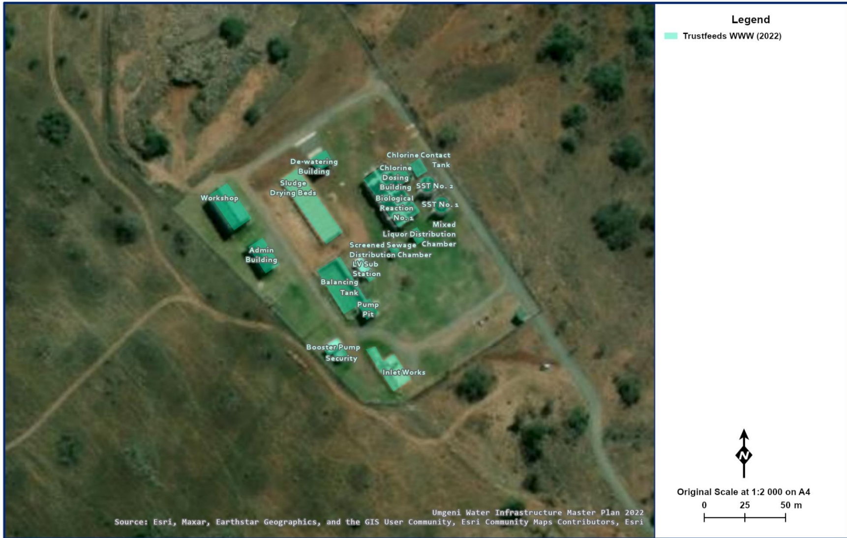
Figure 19.40 Location of Trust Feeds Wastewater Works.
