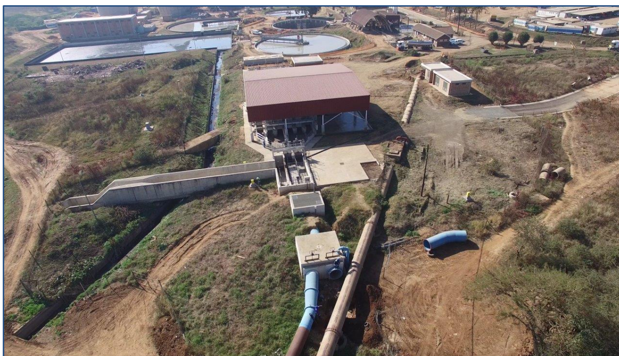
Figure 19.42 New head of works in the foreground with overflow channel teeing-off to the left.
