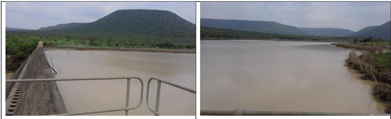
The UTDM appointed a contractor (2018/2019) for the desilting of the Oliphantskop Dam. The impact from the desilting process on water availability is still to be evaluated, but it appears not to have had a positive outcome to improve available yield from the dam.
