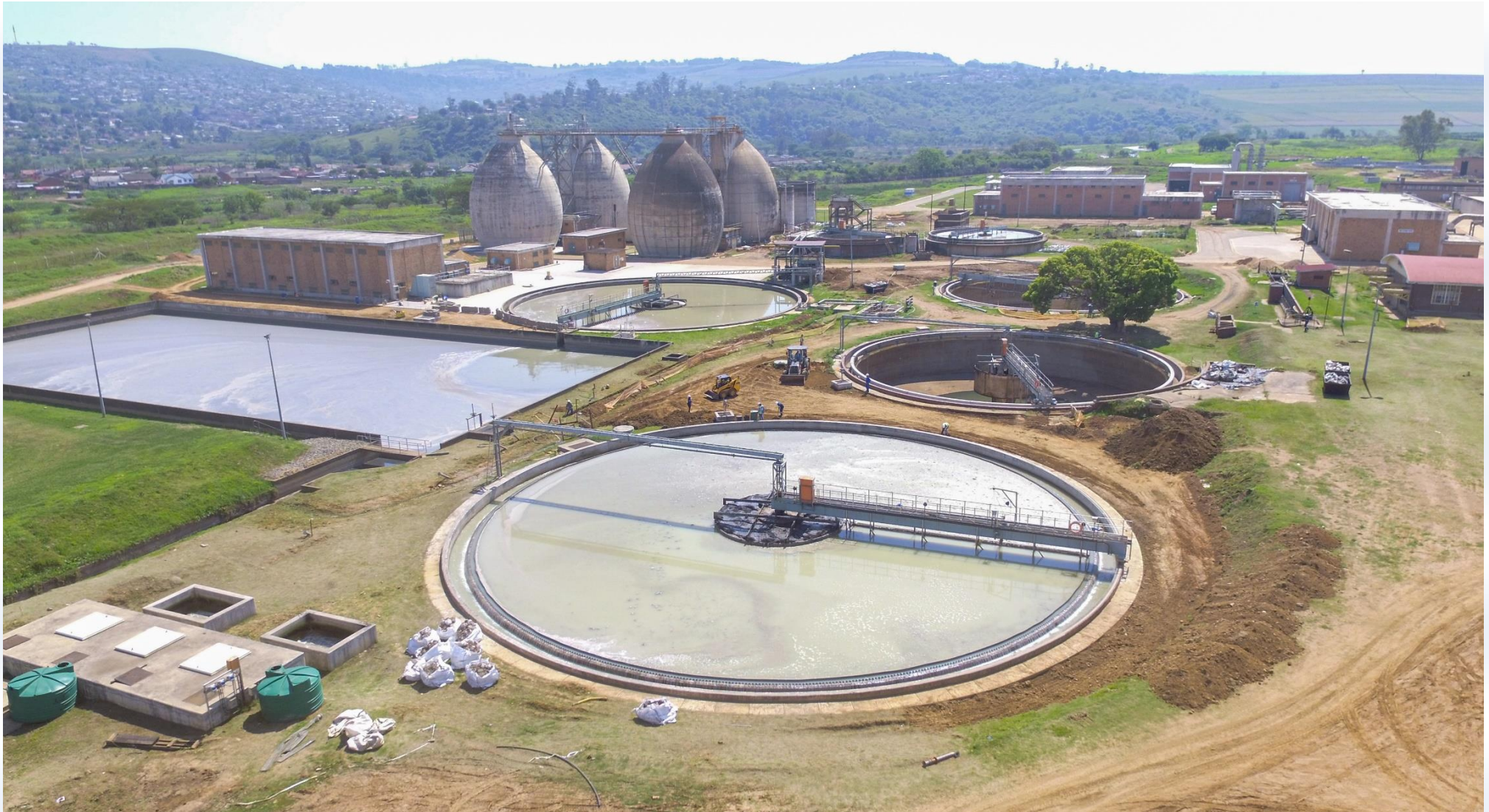
Darvill Wastewater works
