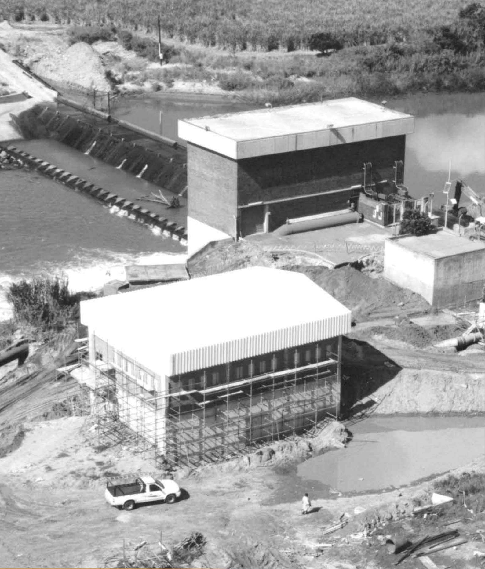
The Mhlathuze Water Weir undergoing an upgrade in 2001.
