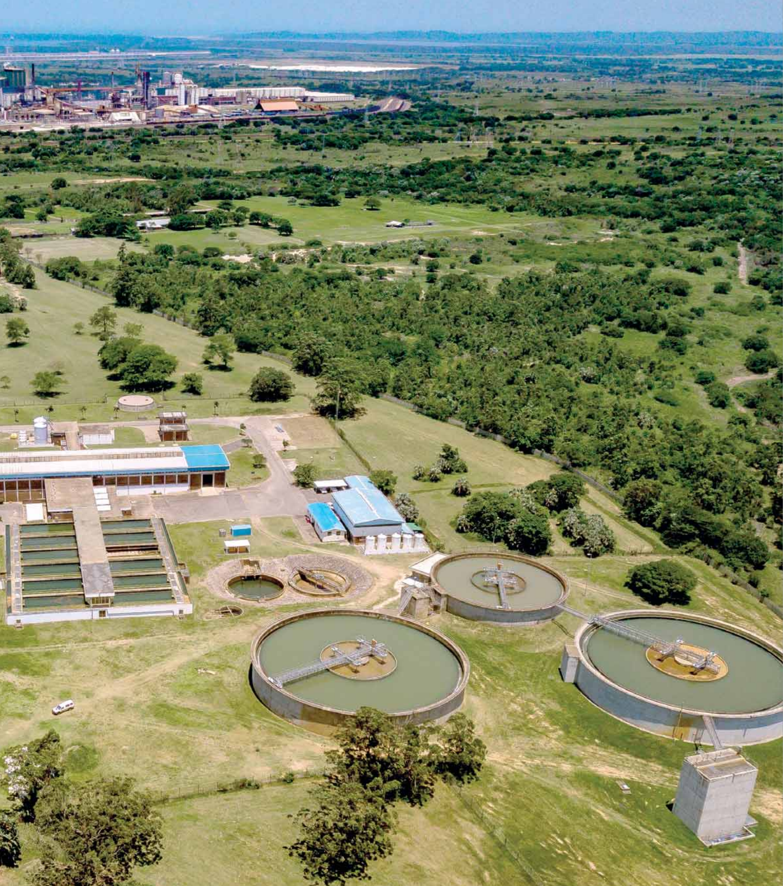
An aerial view of the flagship of Mhlathuze Water, The Nsezi Water Treatment Plant
