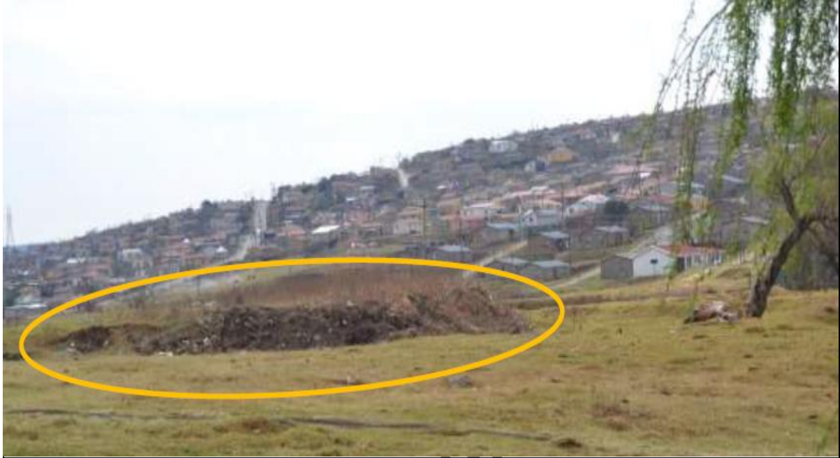
Figure 4: The spoil pile onto which the rock and soil from the excavation was deposited.
